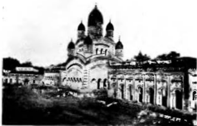
A CORNER OF THE COURTYARD OF THE DAKSHINESWAR TEMPLE, WITH THE TEMPLE OF KALI IN THE MIDDLE.
