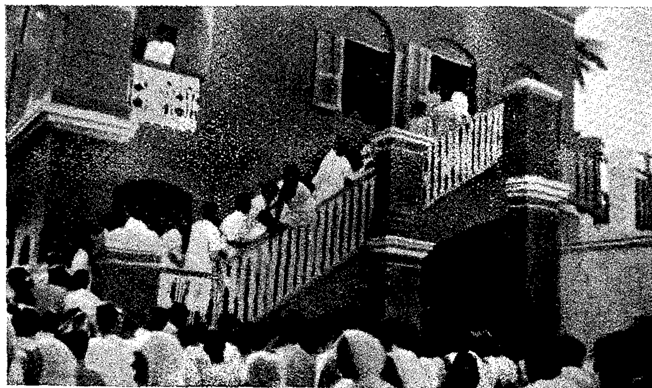
STAIRCASE LEADING TO THE CHAPEL, BELUR
