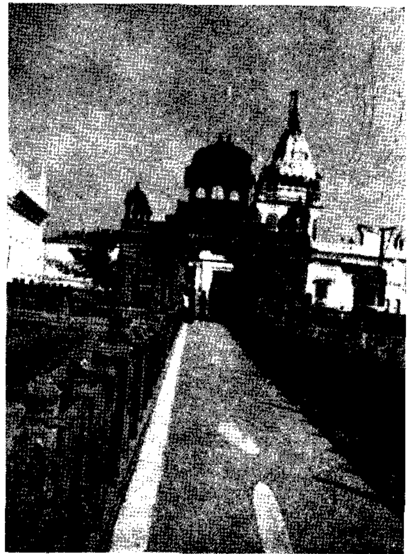
Gateway at the entrance of the bridge (to the Jal Mandir). Behind is the Svetambar Temple
