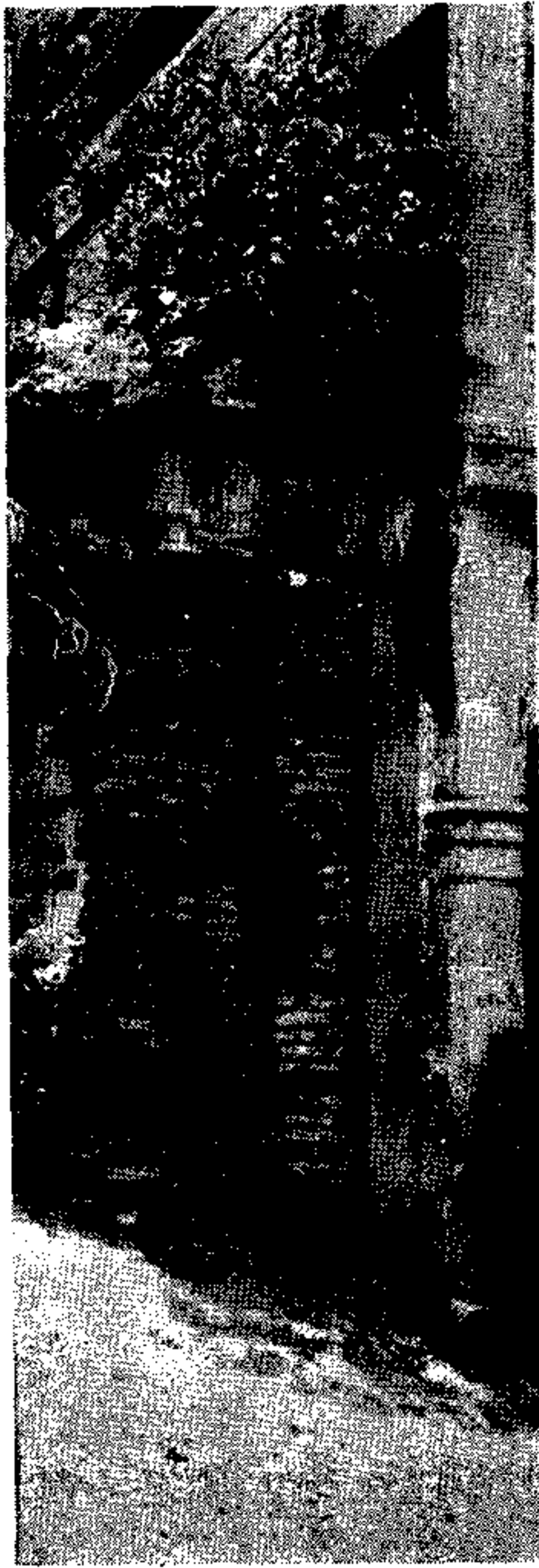
Baranagar Math : ruins of one of the two pillars at the entrance to the old monastery which no longer exists.
