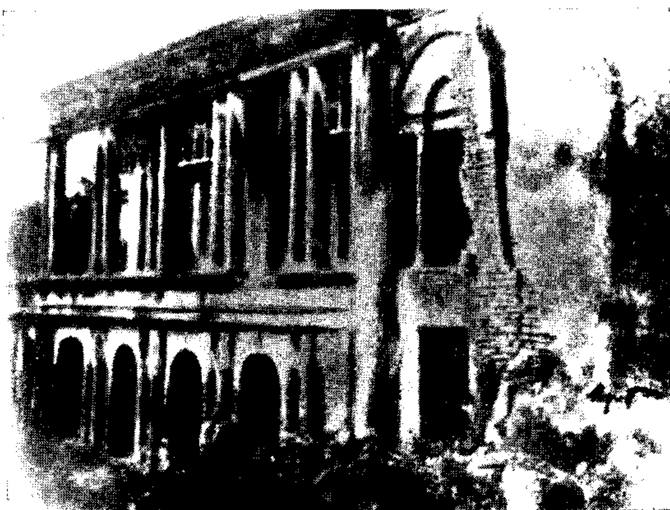
Baranagar Math : the dilapidated building which housed the first monastic community.
