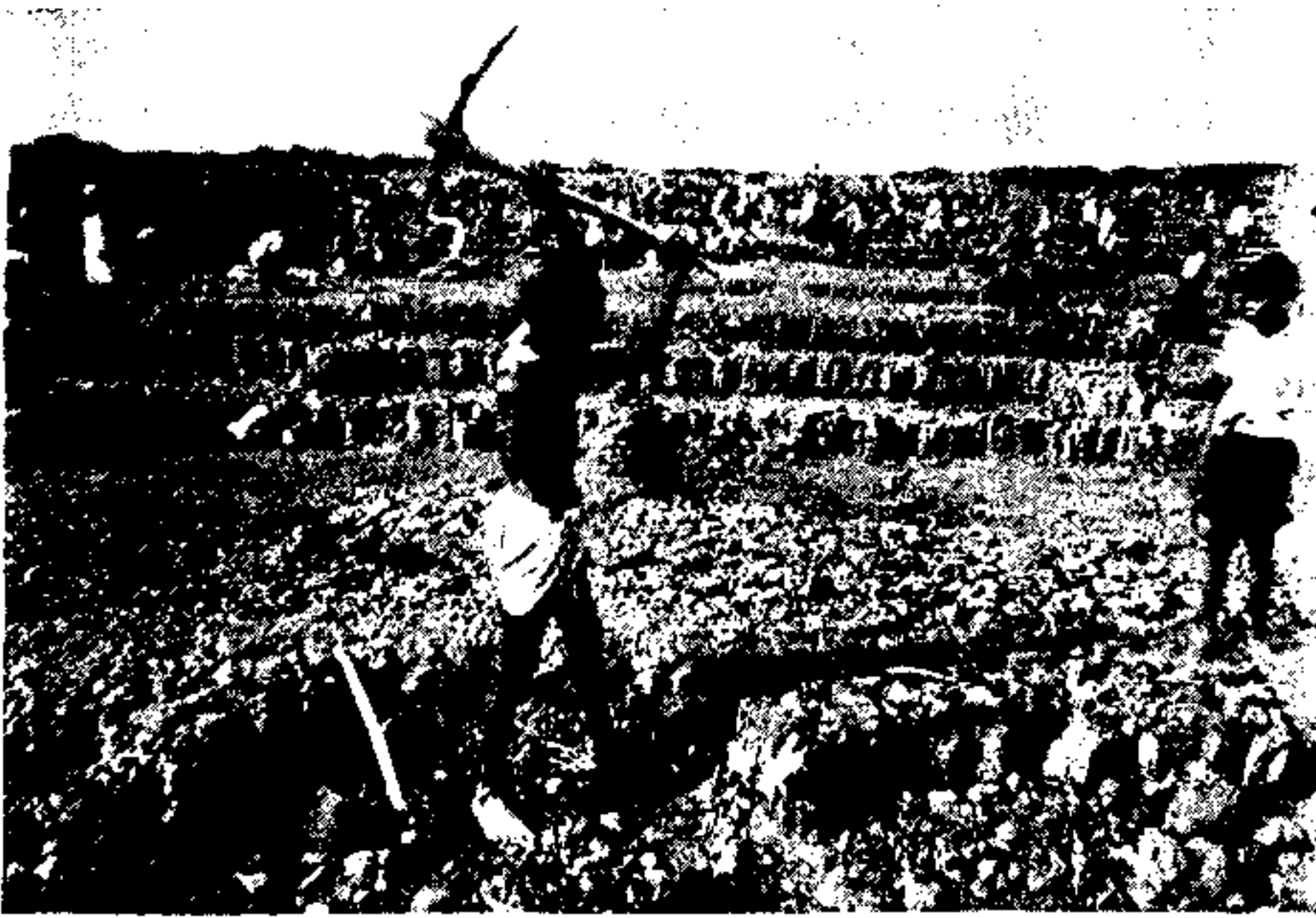
A seven-acre pond being excavated in Gondpendri village, Durg district, Madhya Pradesh
