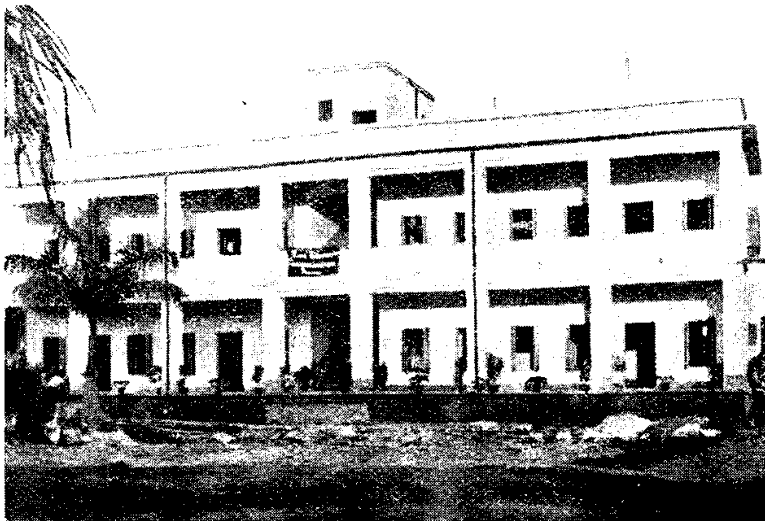
VIDYARTHI BHAVAN, NARAYANGANJ
