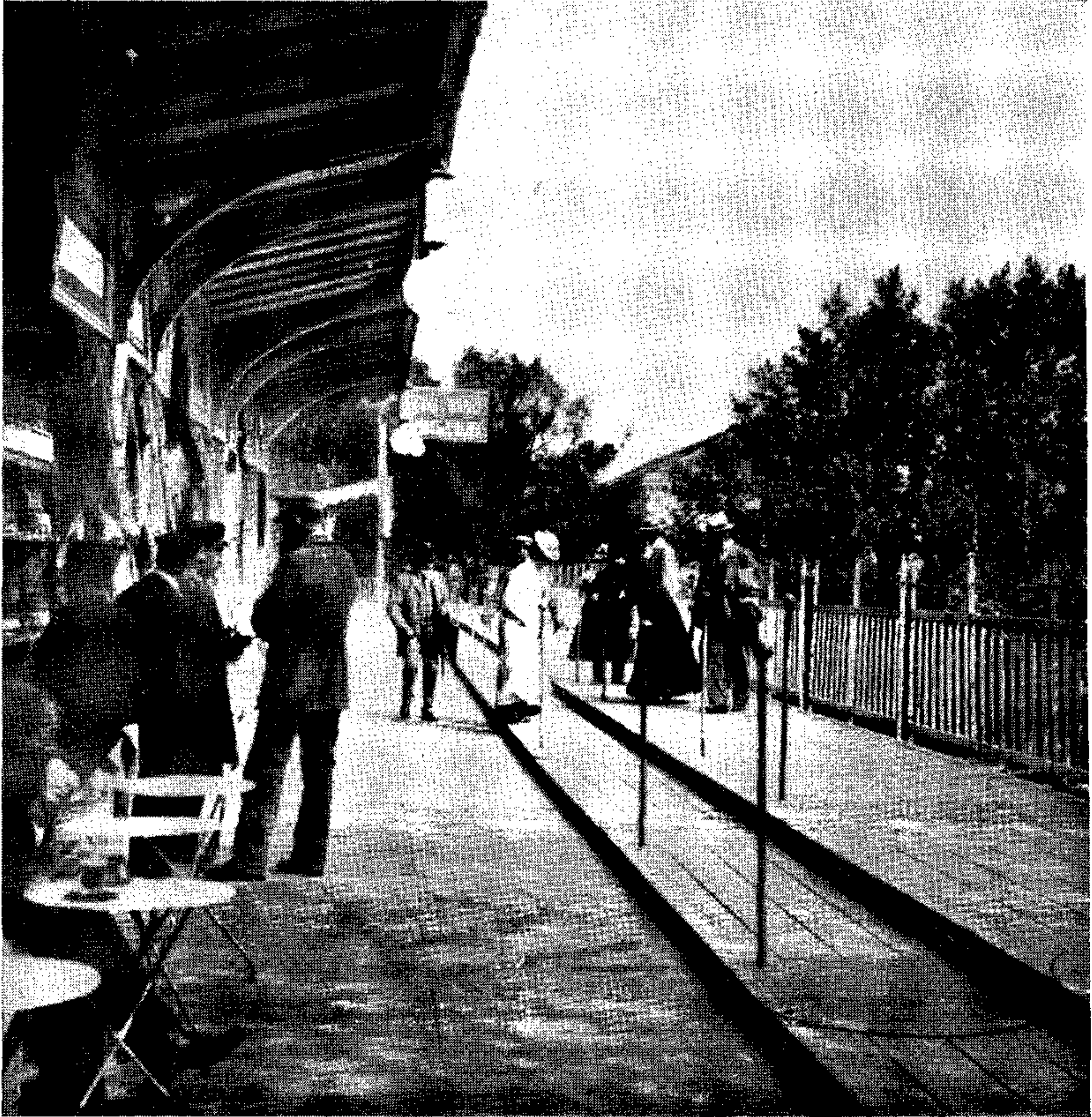
3. Moving sidewalk, Paris Exposition, 1900. The two portions of the sidewalk moved at different speeds, the narrow portion slowly and the wide portion more rapidly. Taking hold of a post to steady himself, the pedestrian stepped first on to the slowly moving strip, thence to the more rapid strip.
